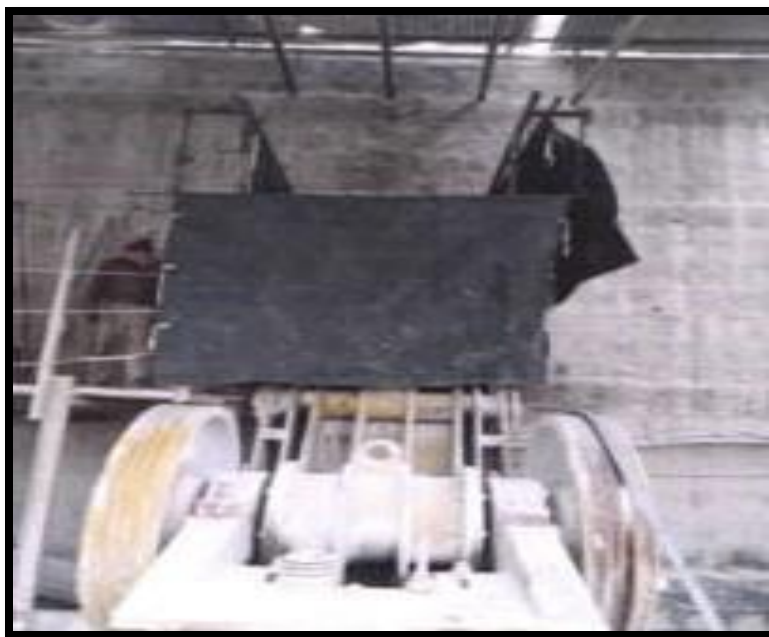
Figure-1: Covering of Primary/Jaw crusher
